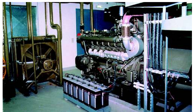
Notstromaggregat
